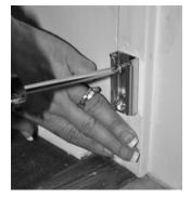
3) Use the screws provided (B), or fasteners of your choice of equal length, to mount the bottom wall mount (D) into the bottom hole locations you just marked (Figure 3). Fasten securely.
