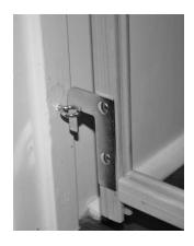
9) Expand the gate and insert the bottom hooking L-bracket on the gate into the bottom screw eye (Figure 13).
