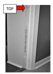
1) Place the mounting template (A) vertically on the wall with "Top" on the template located at the top (Figure 1). The bottom of the template (A) should be touching the floor (it may be convenient to hold the template in place with masking tape).
