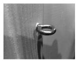
7) Use the screw eyes **(C)** provided and screw them into the hole locations you just drilled **(Figure 8)** installing them flush against the wall.
